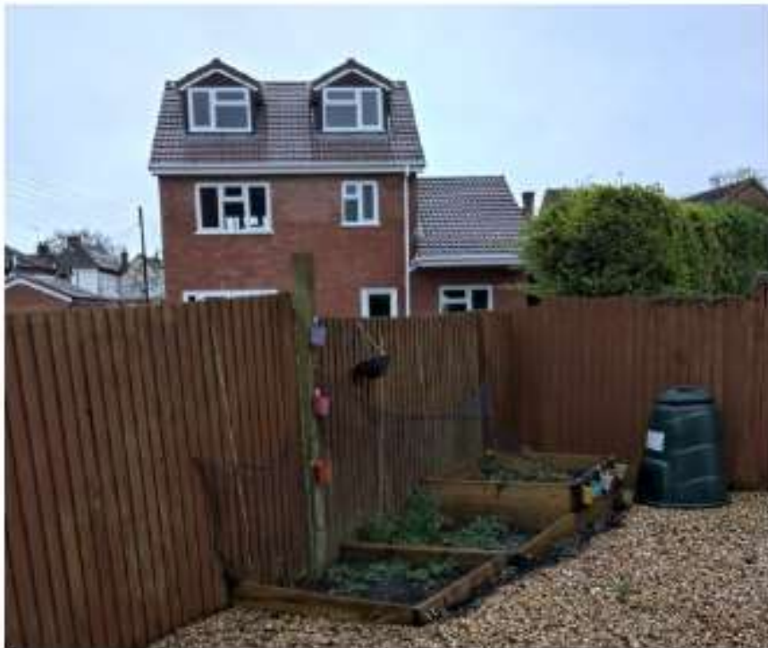
Front of 19 Dellow Grove
